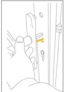
Remove the existing handle from your door (most handles are secured with 2 screws, so remove these). Please note the position of these fixings as you will need to fix your new handles using the existing holes.
